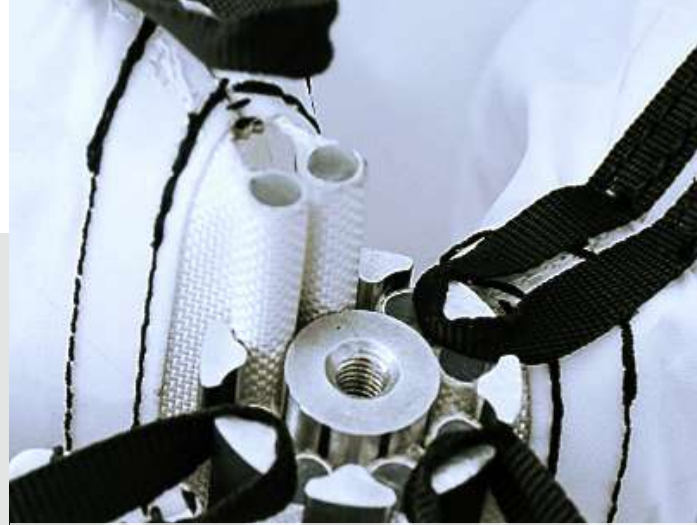
Aluminium keder rail in the tube intersection
